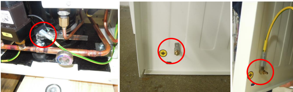
Figure 11: Ground connection details
